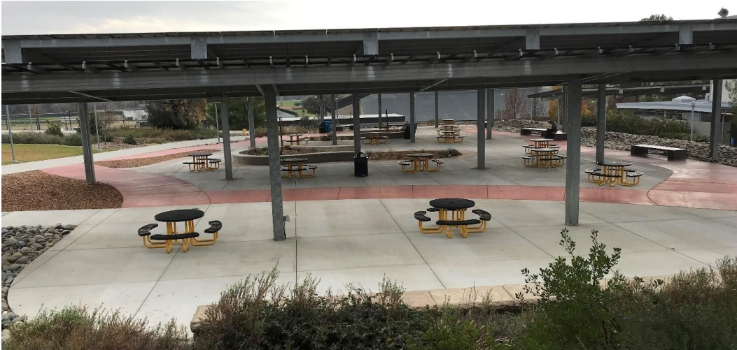
Paved gather area completed by Butte College Heavy Equipment Students
